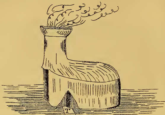
Native smelting furnace at Siddapur.
